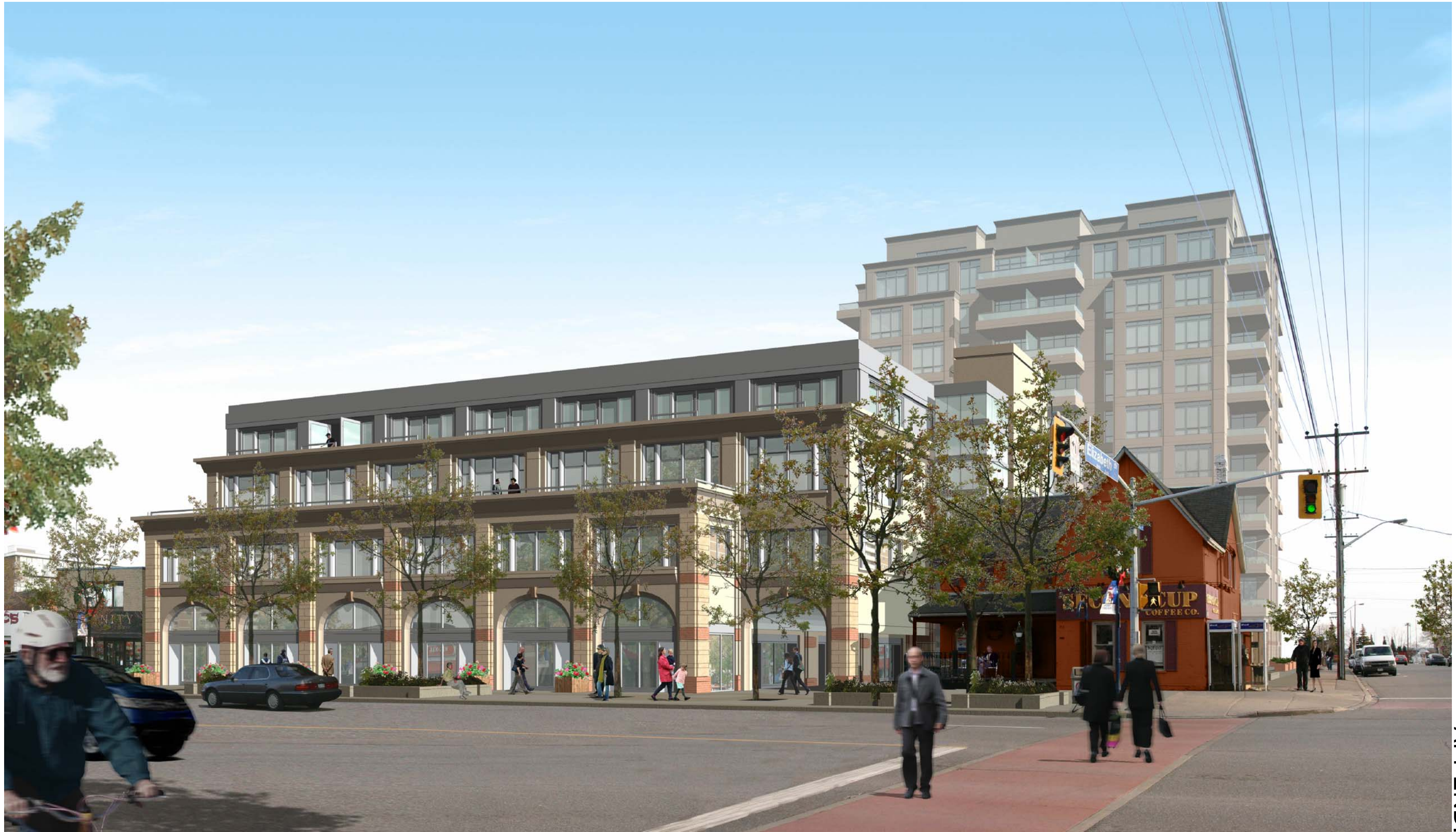
VIEW LOOKING SOUTH EAST
