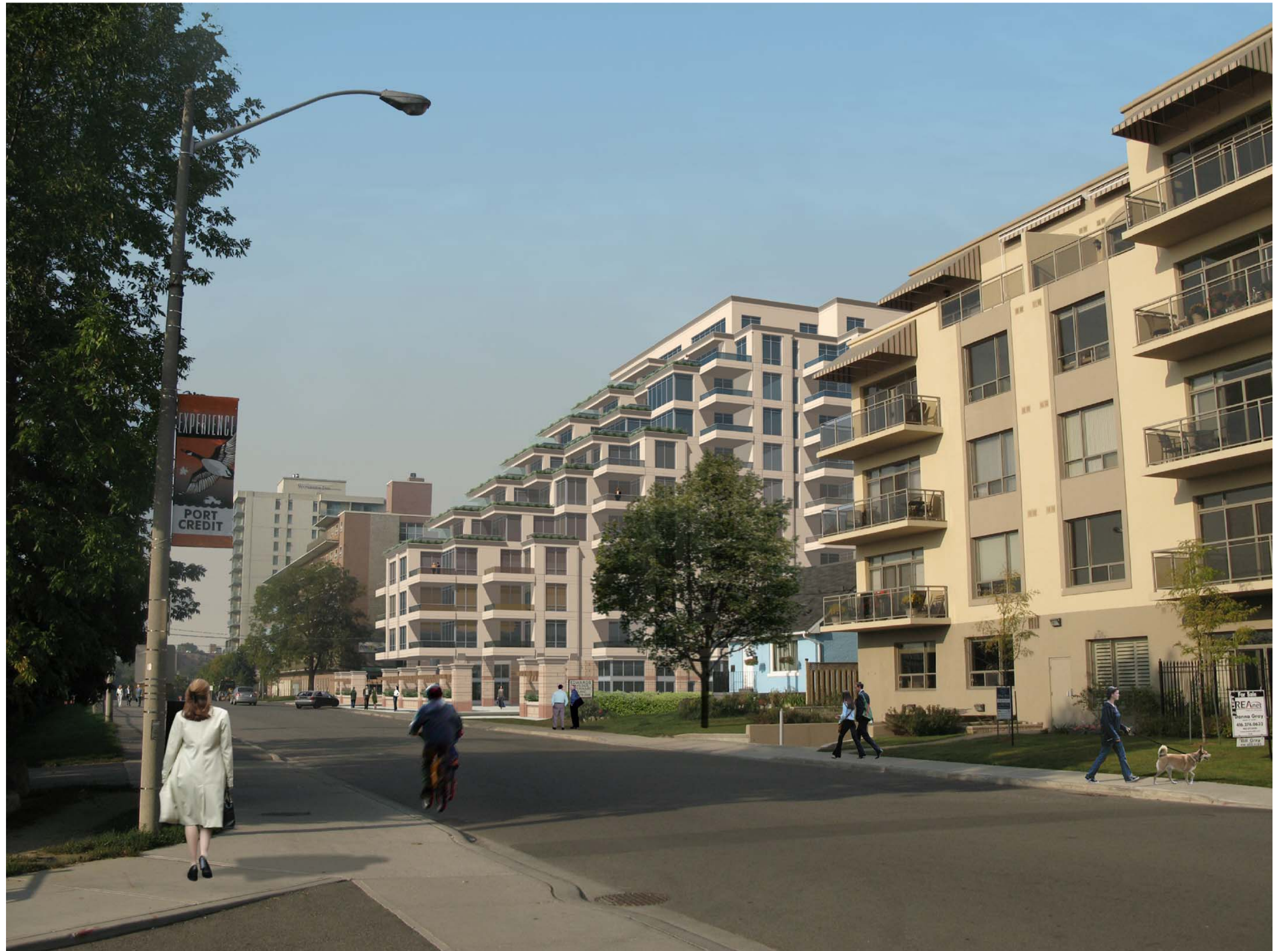
VIEW LOOKING NORTH WEST
